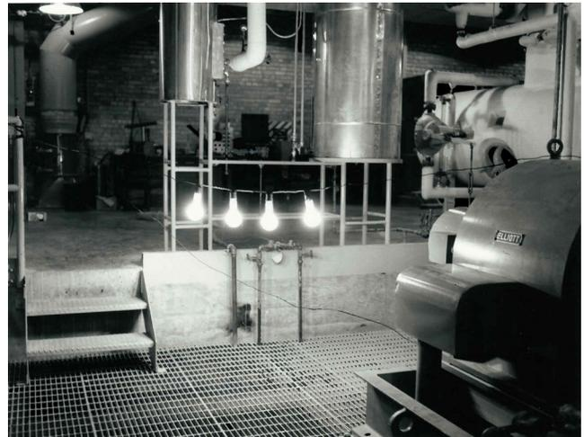
*Argonne's Experimental Breeder Reactor-I in Idaho lit this string of four bulbs with the world's first usable amount of electricity from nuclear power. The date was December 20, 1951.*
